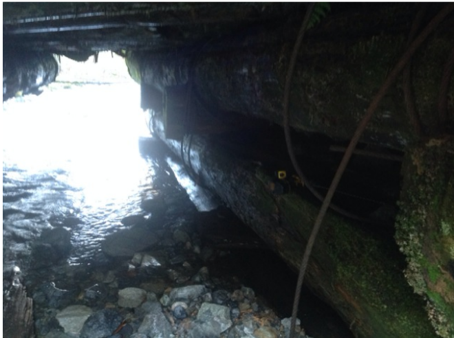
Right Bank Abutment when facing downstream
