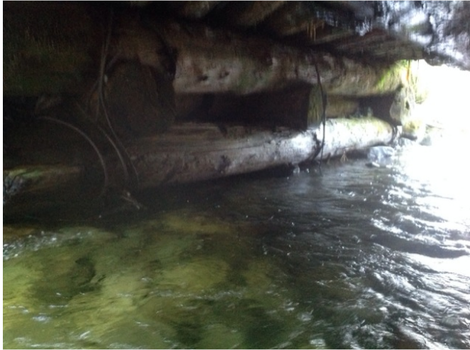
Left Bank Abutment when facing downstream
